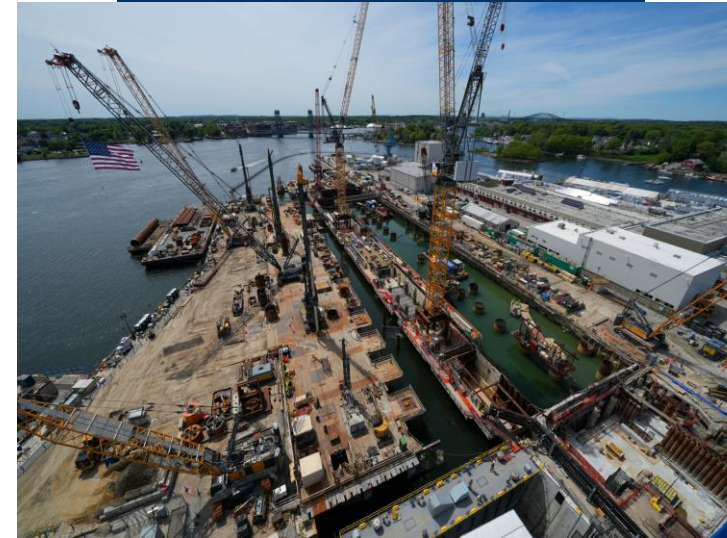
PNSY Dry Dock 1 Expansion
