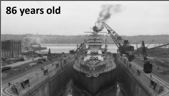
PSNS Dry Dock 4 (ca. 1940)
