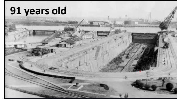
NNSY Dry Dock 3 (ca. 1935)
