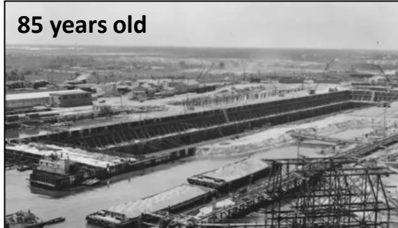
NNSY Dry Dock 8 (ca. 1941)
